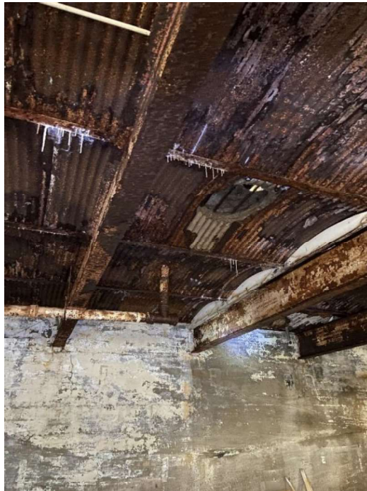
Figure 1 - Steel beams with corrugated metal arches above.
