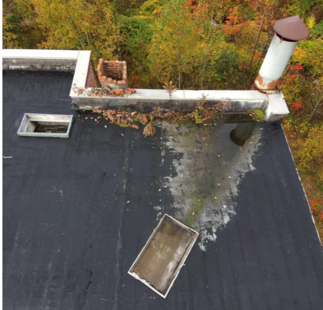
Figure 16 - NW corner of the roof.
