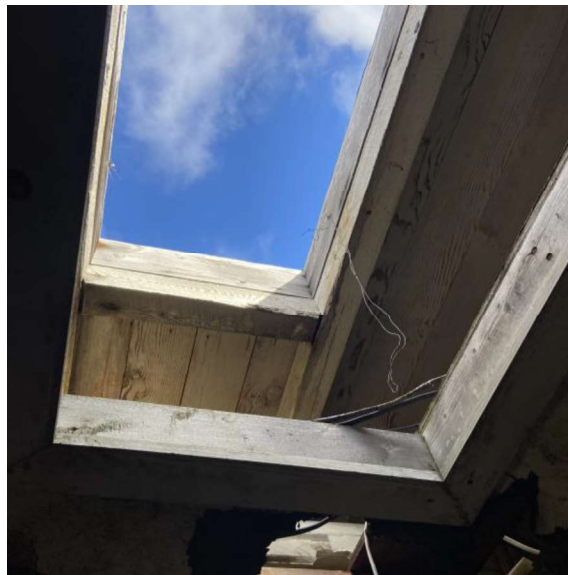
Figure 6 - Roof hatch adjacent to the top of stair at second floor.
